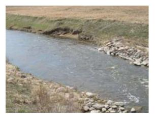
others are just deflecting flow. Instead of guiding the water down the center of the channel, the furthest downstream structure is directing flow toward the opposite bank. This created some extra erosion for a couple years, but it now seems like the bank is becoming more stable and getting a chance to re-vegetate.
